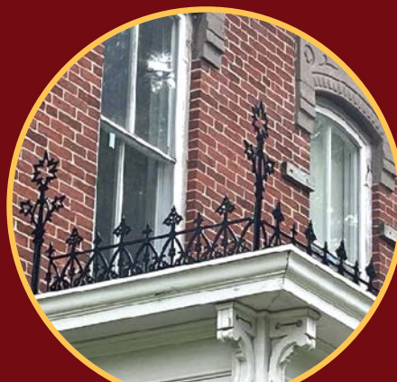
Restored metalwork on Nevada's Briggs Terrace-Evergreen Lane house.
